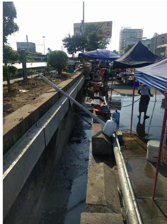
Figure A.18: At the south side of Strand Road there was a sharp increase in the ground level elevation. Here a road referred to as Raised Strand Road (see Figure A.13, officially also called Strand Road), was elevated and used for trucks to transport containers to the various Yangon Port terminals. The elevation difference was around 2 meters. Therefore the raised Strand Road acted as a sort of large dike, separating the Latha Township and the Yangon River. View from the south side of Strand Road, looking to the west. Left the Raised Strand Road, right Strand Road. In the middle an open drain that runned along the south side of Strand Road, see Figure C.11. Picture taken on March 19, 2017.
