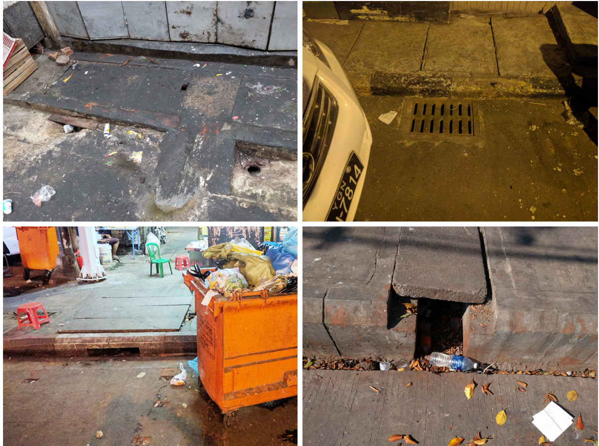
Figure C.9: Example of four different drain inlets. Top left: small pipe like holes on 18th Street upper block. Top right: grated inlet on 18th Street lower block. Bottom left: large rectangular inlet on Latha Street. Bottom right: square inlet on Strand Road. The drain could be seen as canal from concrete or brick and mortar walls, covered by concrete slabs. The type of inlets, state of maintenance is varying from location to location. All pictures taken between 28-02-2017 and 05-03-2017.
