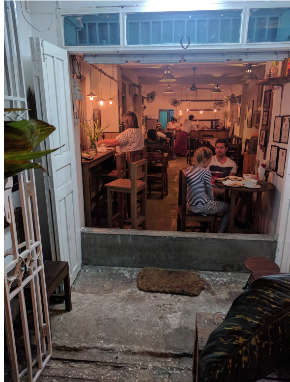
(b) This was an example of the a building with flood protection. The concrete slab also functions to keep out rats. Picture taken on January 21, 2017.
