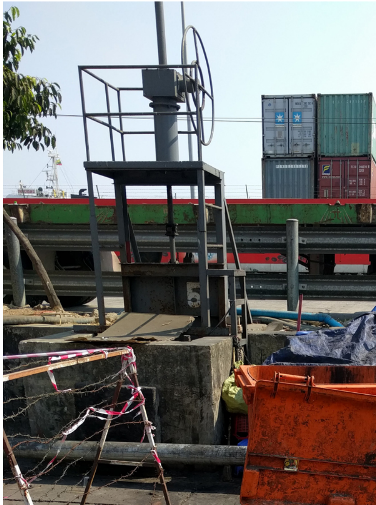
Figure 3.6: Flood gate structure (FGS 6) along Strand Road. Picture taken on March 19, 2017.
