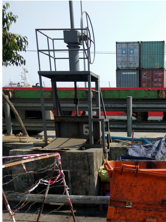
Figure C.19: Flood gate structure along Strand Road.
