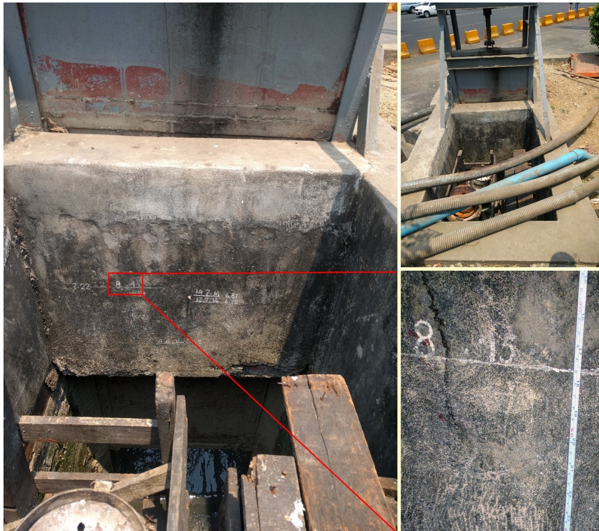
Figure C.15: Scratch marks made by employees of YCDC EDRB for flood records. The scratch marks were on the inside of the FGS, downstream of the gate (for the normal drainage direction). Left you see the inside of the FGS. The top right provides an overview. Details of one of the flood mark records are shown bottom right, with own measurements to relate the measurements from YCDC to ground levels. All photos were taken on 06-04-2017.
