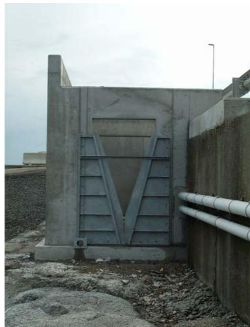
**Fig. 14:** *Compound weir (seen from outside the overtopping tank).*
