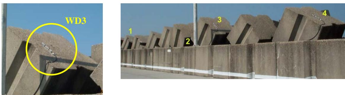
**Fig. 23:** Wave detectors (WD); detail (WD3) and situation (4 of the 6 detectors)
