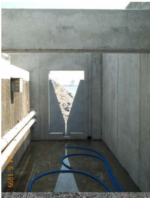
**Fig. 13:** *Compound weir (seen from inside the overtopping tank)*
