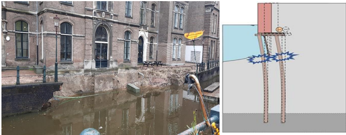
Figure 1.1. Collapsed Grimburgwal 2020 and failure mechanism wooden piles (TUDelft.nl)
