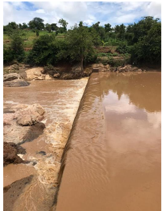
Figure 5 Sand storage dam during wet season.
