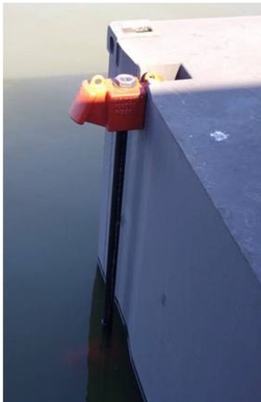
Figure 1.6: A representation and schematic of the connection between a DMB and coupling [1]
