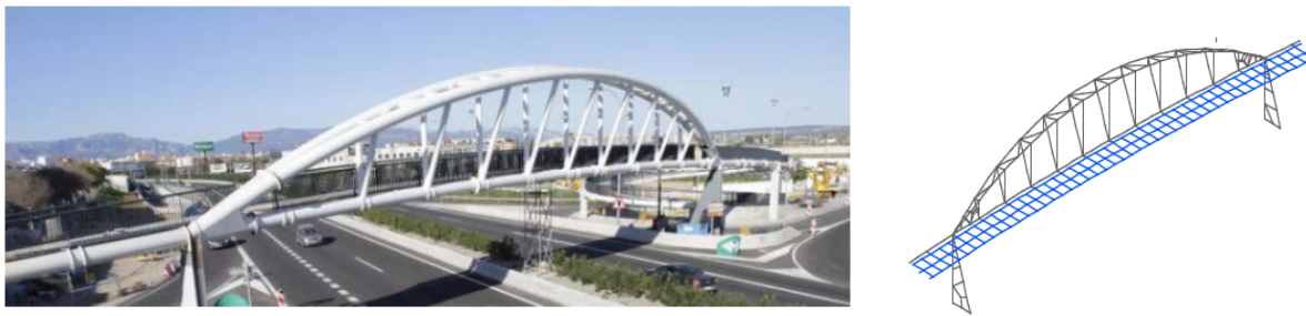
Figure G.1: Footbridge under study: Photograph and numerical FE model [16]
