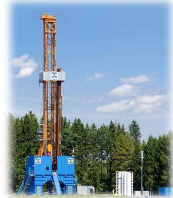
Figure 2.3 An image of a geothermal drilling rig during the construction. To reach the 70 C water well at depth of 2.1 km extensive drilling is required (Source: Energieoverheid, 2016).
