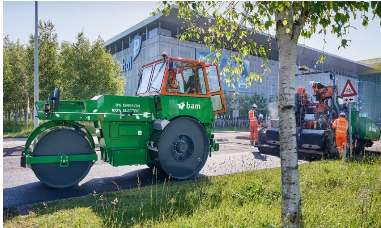
Figure 26: SMA with electric roller
