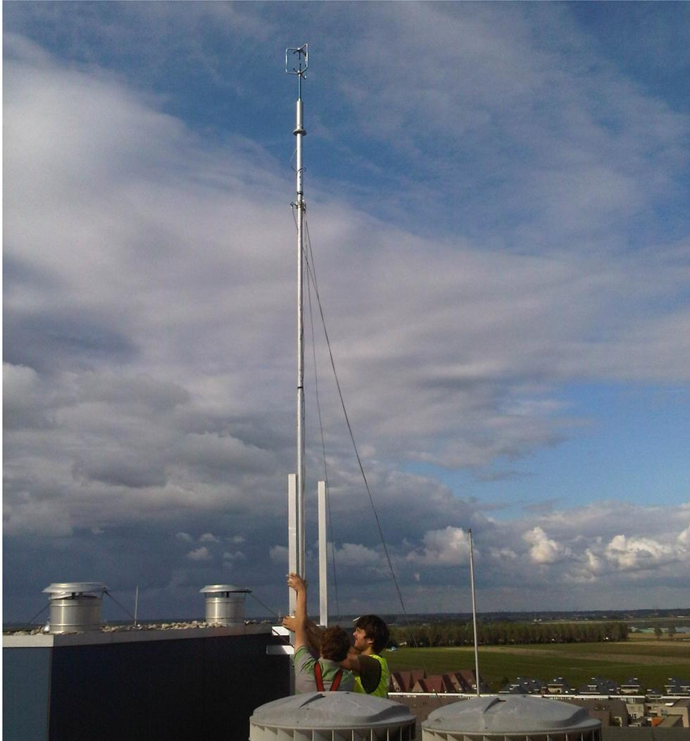
Figure D.4: Mast installation in August 2011 on the Witte Dame. Here shown is the 6 m setup, which was later extended to 7.3 m.
