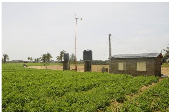
Figure 60. Renewable energies at Tip Top Farms. The wind turbine (middle) and PV cells (roof) power the pumping system for which water is stored in the black tanks on the roof. The wiring of all the technologies is housed in the shed.
