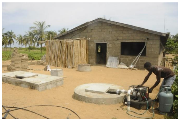
Figure 59. The biogas digester at Tip Top farms.
