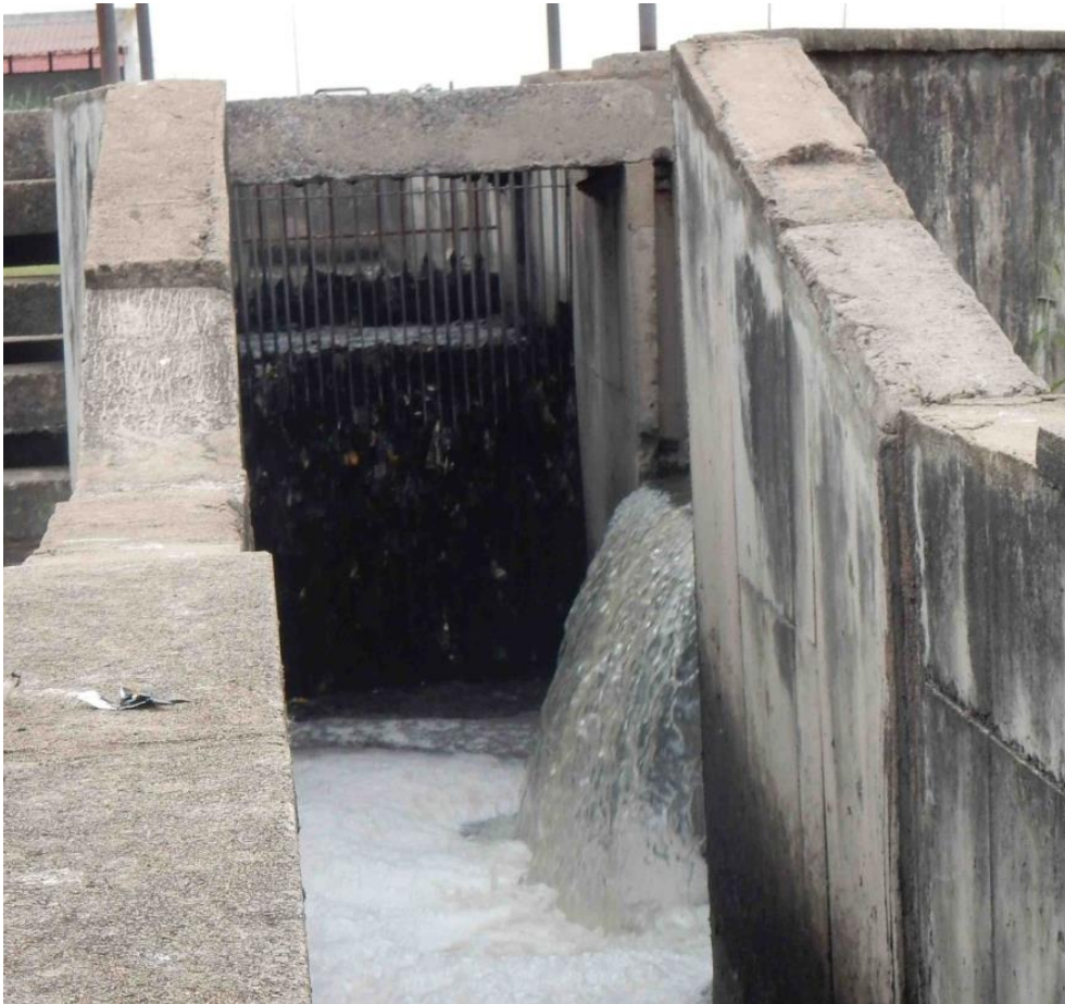
Figure 11: Photo of bar-screen at the entrance of the WWTP. Since the screen is clogged by debries, the water by-passes the screen through the over-flow.
