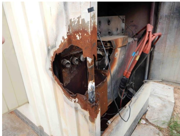
Figure 9: Meltdown of electrical system of pumping station two.
