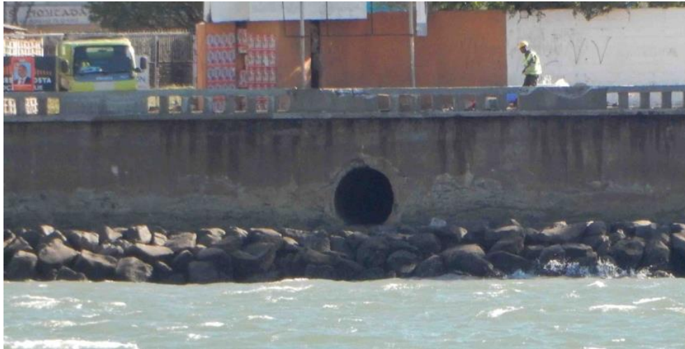
Figure 13: Discharge of untreated sewer into the bay.
