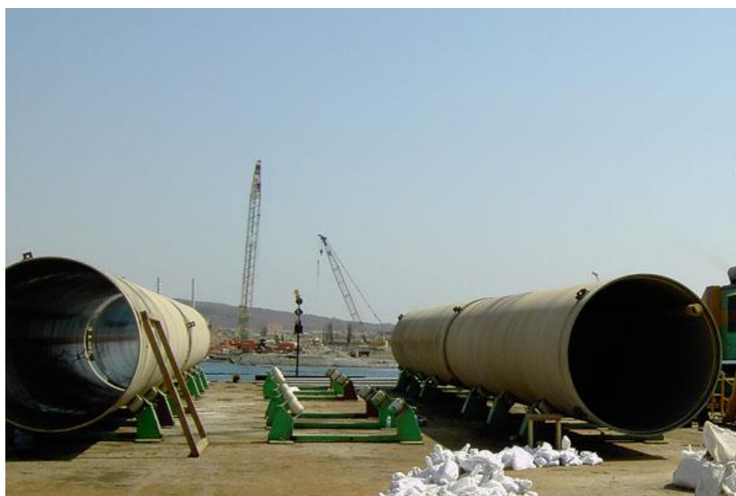
Figure 14: Preparing FRP pipes for installation
