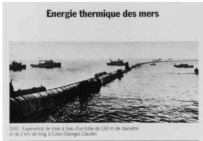
Figure 4:Deployment of Claude's Cold Water Pipe
