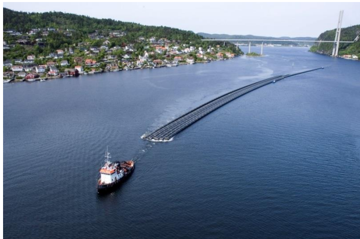
Figure 11: Transport of HDPE Pipe Segments
