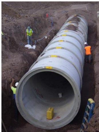
Figure 15: Connecting Concrete Pipe Segments
