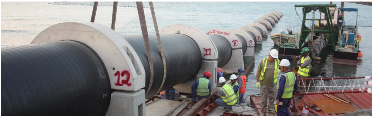
Figure 10: Installation of a ballasted HDPE Pipe
