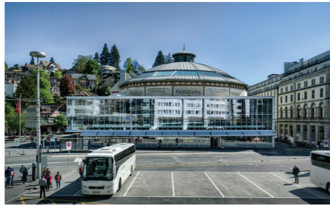
Fig. 70. photo of the Bourbaki-Panorama building in Luzern, Switzerland (Kümmerli, 2017)
