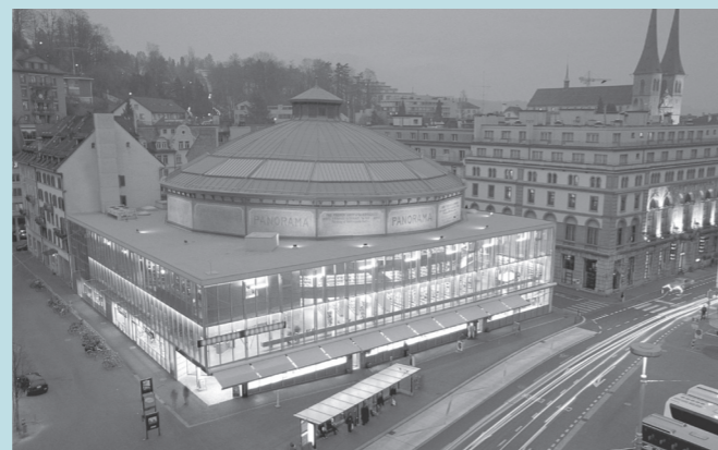
Fig. 7. photo of the Bourbaki-Panorama building in Luzern, Switzerland (Kümmerli, 2017).
