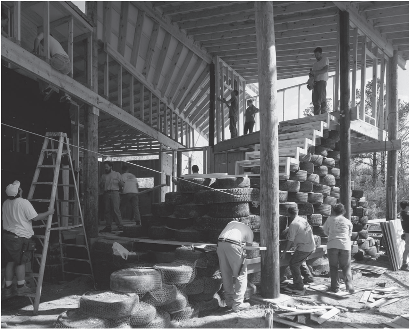
7.8 Rural Studio, constructing the Shiles House , Hale County (AL), USA, 2002
