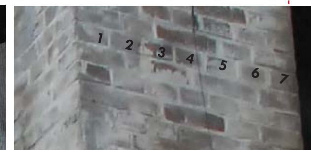
7x head brick = (7x100 + 6x12) 770 mm
