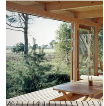
Glass sliding doors in timber frame
