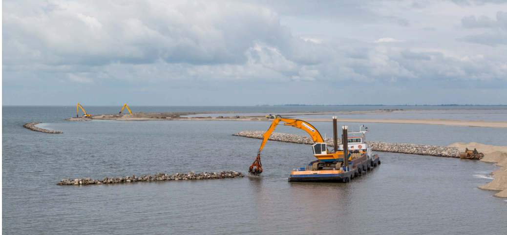
Figure 5. Dredging techniques, via paansvanoord.com 2
