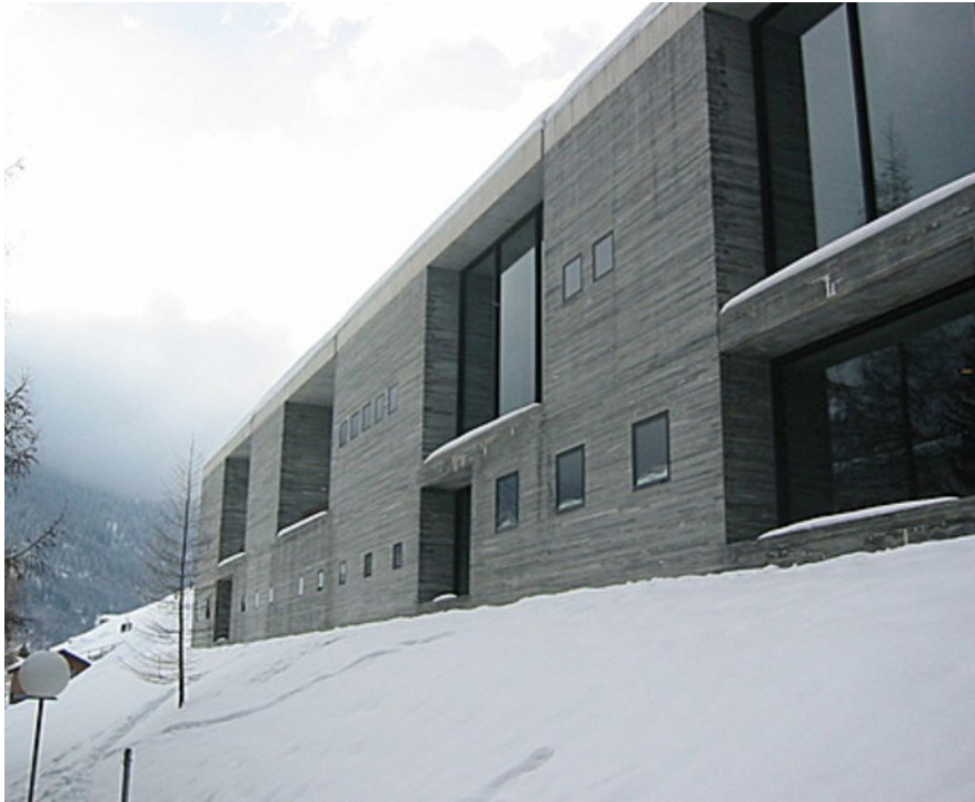
Architects: Peter Zumthor, with Marc Loeliger, Thomas Durisch and Rainer Weitschies Location: Graubünden, Switzerland Project Year: 1996
