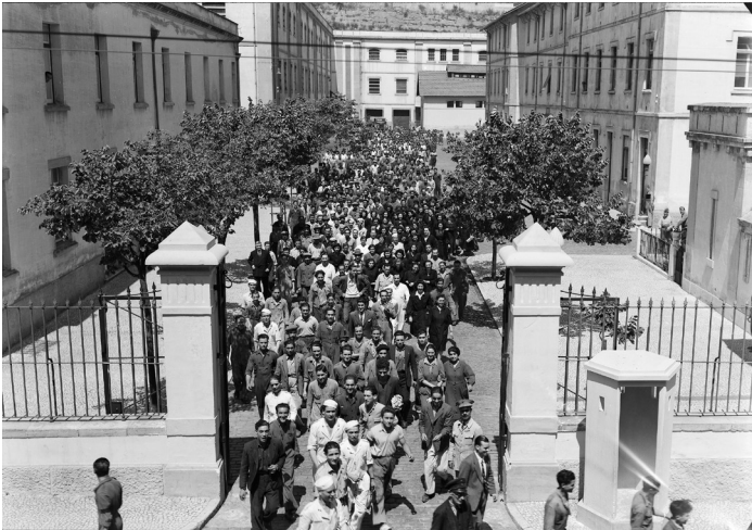
Image 42: Workers of the MMC (DOCOMOMO Archive photographical survey)
