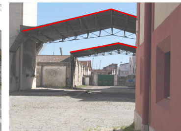
Image 36-37: A connective element ending in a silo (showing that it was used for products) and additional roof structures (Groupwork Cultural Value p.9)
