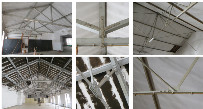
Image 69 t/m 74: Wooden and steel trusses with different details
