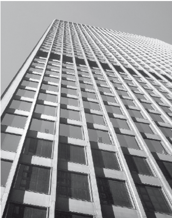
Curtain wall, federal center Chicago (Knaack et al., 2007)
