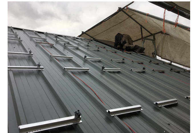
Figure B.5: Roof, installation solar panels (B.I.K Bouw, 2018)
