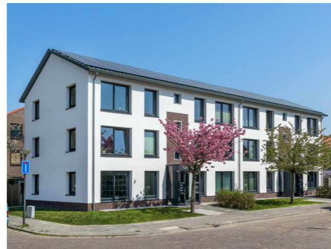
Figure B.1: 2ndskin demonstrator front façade (B.I.K Bouw, 2018)
