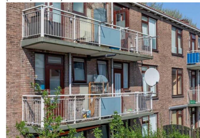
Figure B.6: rear façade, before the renovation (B.I.K Bouw, 2018)
