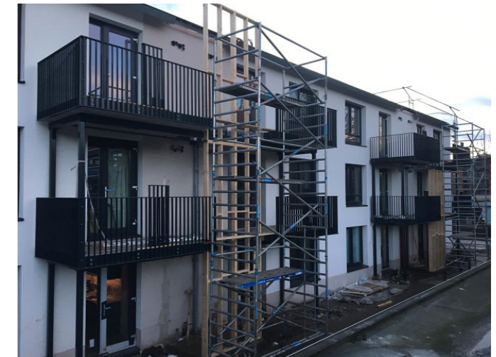
Figure 5.16: Building the cupboard (B.I.K Bouw, 2018)
