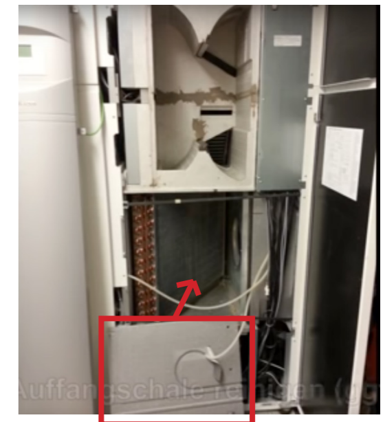
Figure 5.23: open module LWZ model (Stiebel Eltron, 2016b)
