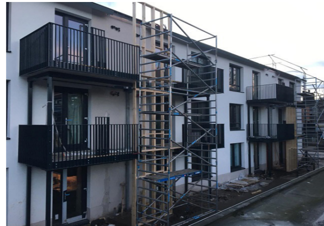
Figure B.8: rear façade, before the renovation (B.I.K Bouw, 2018)
