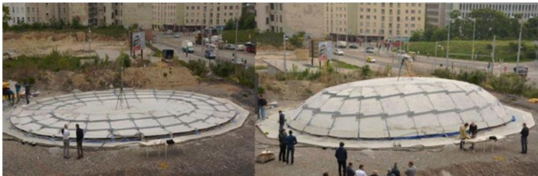
Illustration 3.3: The plane concrete plate is produced and the membrane is inflated [10]
