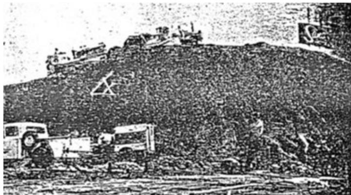
Illustration 3.4: Forming soil mould for concrete shell [8]
