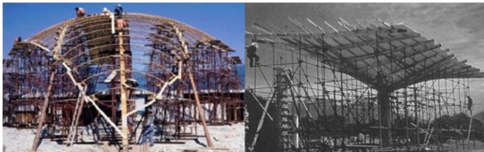
Illustration 3.2: Examples of elaborated timber formwork for concrete shells[9], [25]
