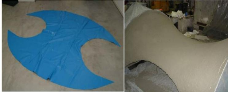
Text 1: Fabric formwork and the resulting panel [24],
