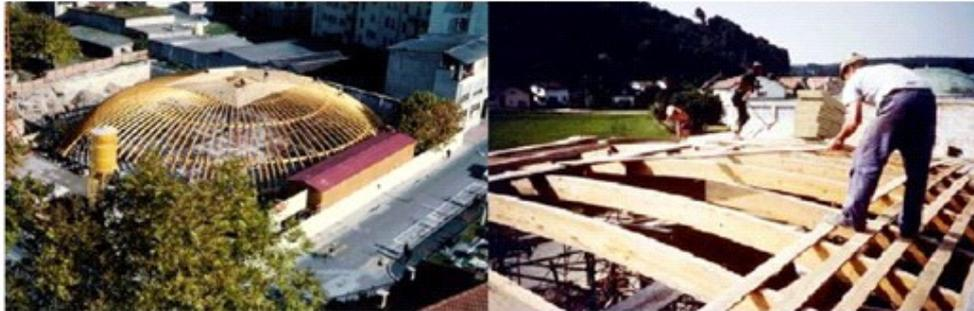
Illustration 3.1: Shapes, formwork and skeleton shuttering[9]
