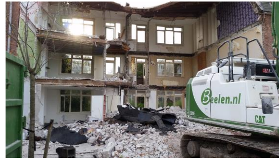
Figure 37. Recent demolition of apartments at the Schilderswijk.
