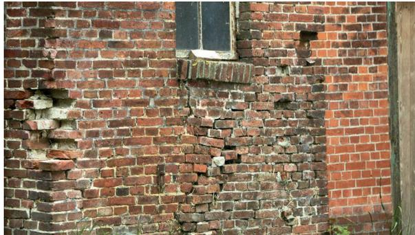
Figure 1.2: A house destroyed due to surface subsidence in Groningen. This figure is retrieved from [19].
