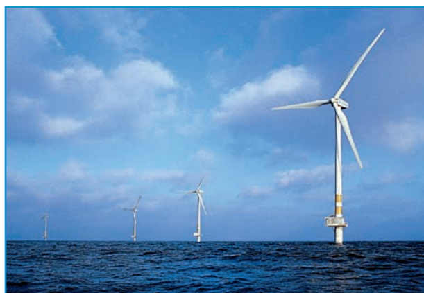
figure 5. Utgrunden off-shore wind farm, consisting of seven 1.5-MW wind turbines erected for the Swedish coast. (Courtesy: GE Wind Energy.)
