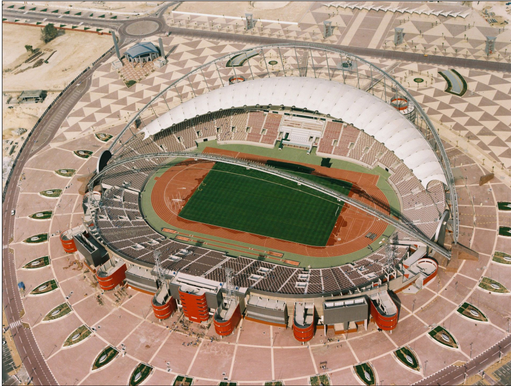
Fig. 3: Current situation Khalifa International Stadium (Legacy, 2016)
