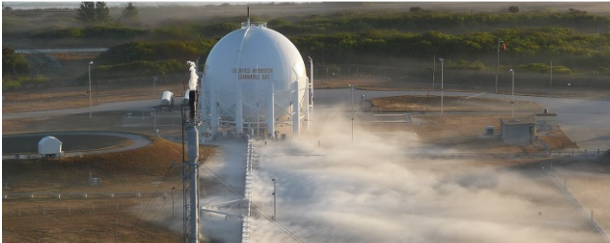
Figure 1.3: Boil-off trail during the ground storage of liquid hydrogen.
