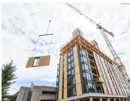
Figure 2.5: Tall wood building, UBC Brock Commons Vancouver (Pilon et al., 2016)
