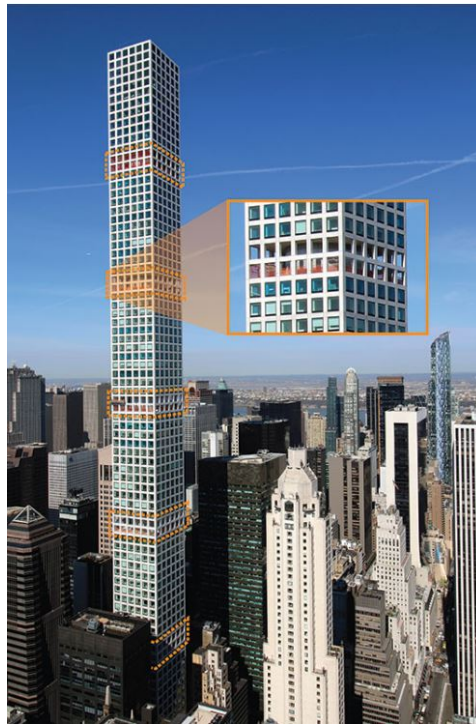
Figure 7.23: 432 Park Avenue with double story openings at five levels (Galsworthy et al., 2016).
