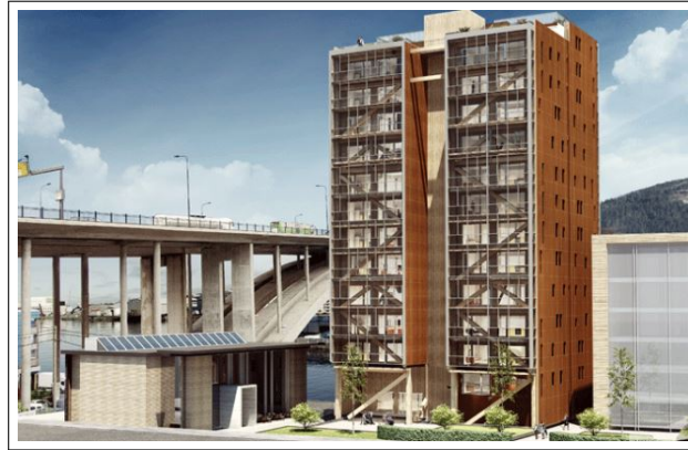
Figure 2.12: Treet building in Norway (Abrahamsen and Malo, 2014).
