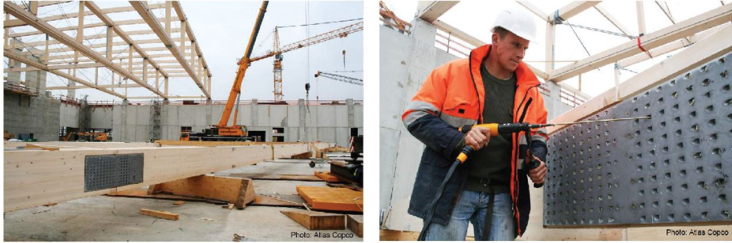
Figure 2.21: Large timber screw connection in truss (Blass, 2010).
