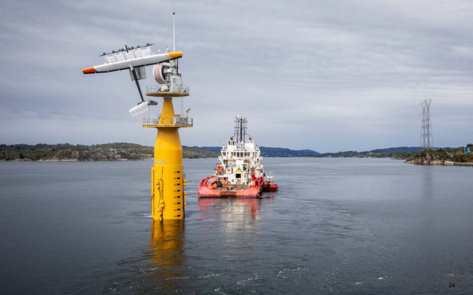
Makani's kite and floating platform were towed offshore by two coastal tugboats (31 July 2019)
