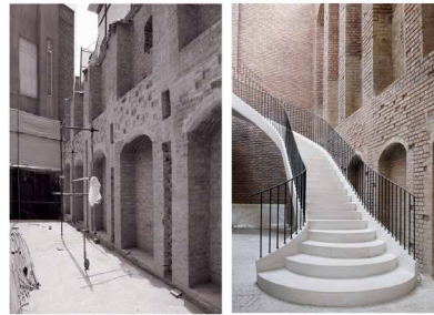
Argo Factory, before and after adaptive reuse (ASA North, Archdaily webpage: https://rb.gy/oxanfj )
