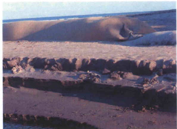
Figure 8-2 Dune care in the north of Waihi Beach and a sand sausage to trail Waihi Beach Stream
