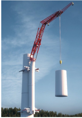
Figure 9.1: The Lagerwey self climbing crane [39].
