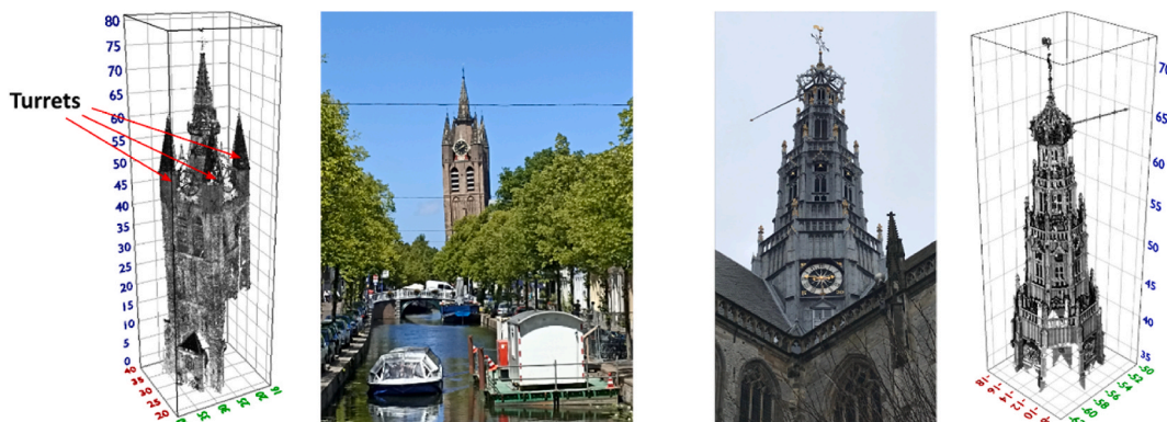
Fig. 1. The Old Church in Delft (left panels), and the St. Bavo's Church in Haarlem (right panels) tower pictures and point clouds.
