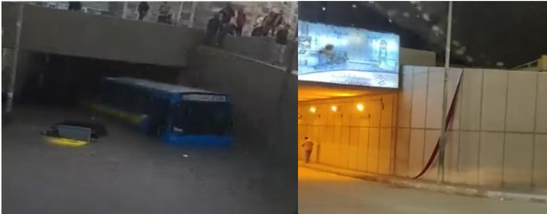
Figure 2.7 Many hotspots are in tunnels (tunnel exit), Nov 20 2021 Source: ( YouTube: Chave Weather-daily videos )(left) Hose at the same location. Tunnel entrance (right).
