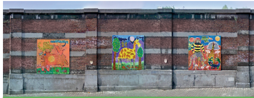
Collage of the facade with the art project of kids on it
