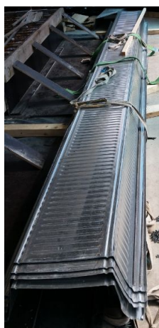
(a) A pile of steel decks
