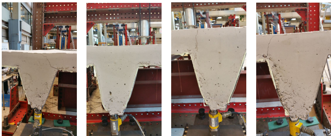
(a) End of the rib at location E5 (see figure 7.38). (b) End of the rib at location E4 (see figure 7.38). (c) End of the rib at location E2 (see figure 7.38). (d) End of the rib at location E1 (see figure 7.38).
