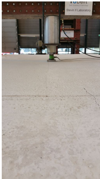
(a) Longitudinal crack alongside rib 3.
