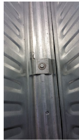
(c) A connection at bottom rib
