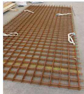
(b) The reinforcement meshes of \text{Ø}8-150
