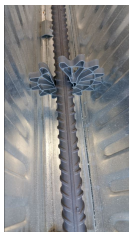
(a) Bottom reinforcement bar in a rib
