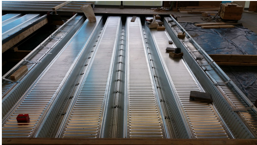
Figure 7.9: The connected steel decks, constructed out of five single deck elements
