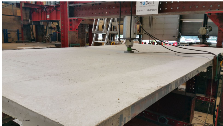
(b) Longitudinal crack alongside rib 3.
