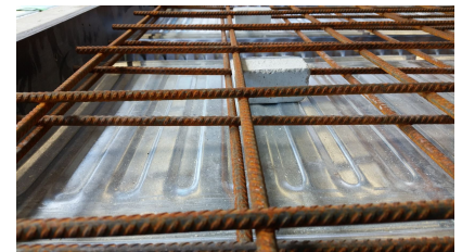
(c) Top and bottom mesh reinforcement
