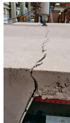
(c) Detail of the longitudinal crack alongside rib 3.
