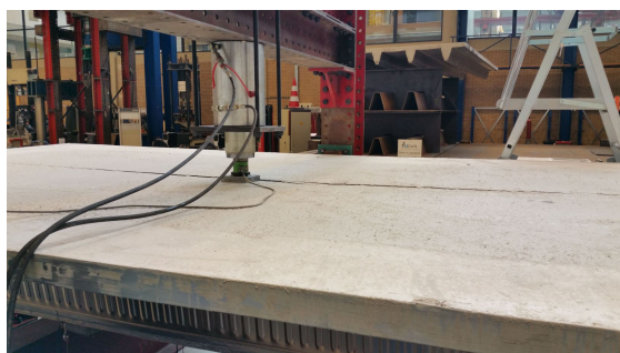
(a) Longitudinal crack alongside rib 3.
