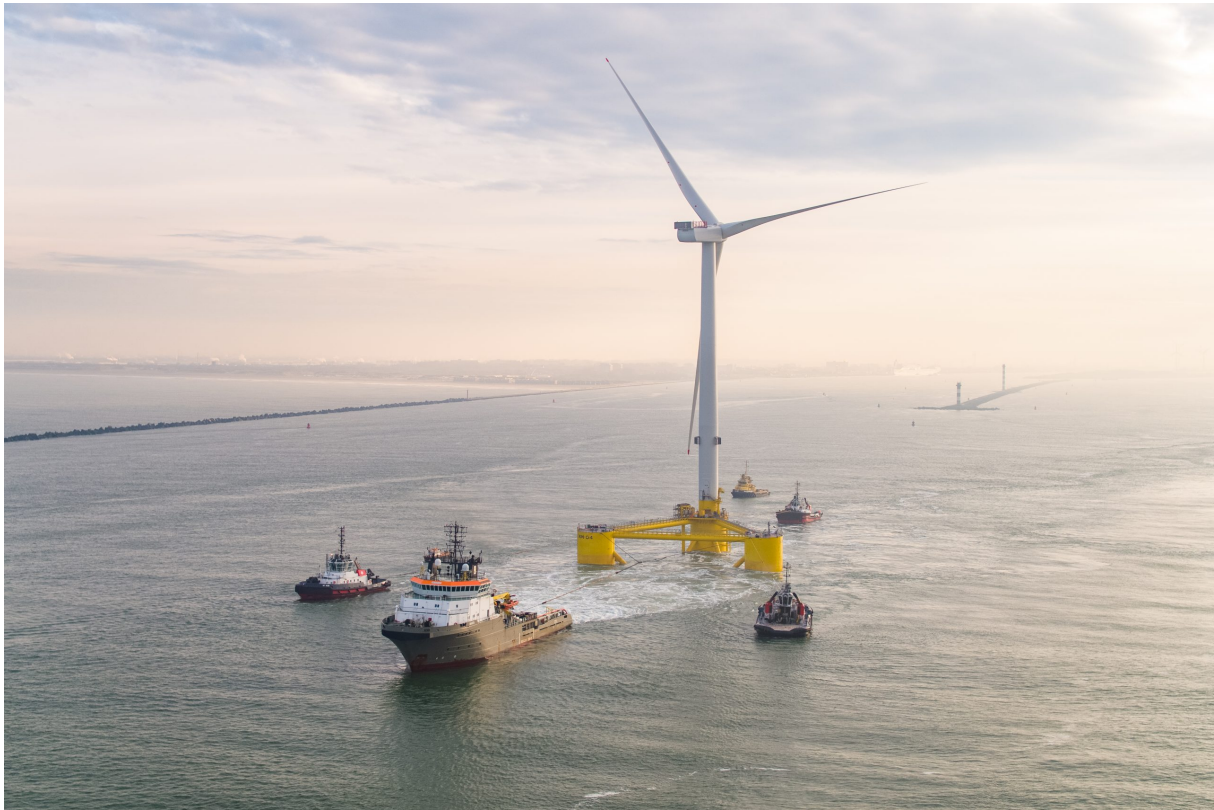
Figure 1.2: Tow of a complete wind turbine on a semi-submersible sub-structure [33].
