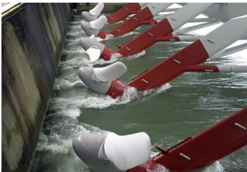
FIGURE 24: TOCARDO IN-SHORE TIDAL TURBINES INSTALLED AT EASTERN SCHELDT [WWW.TOCARDO.NL].
