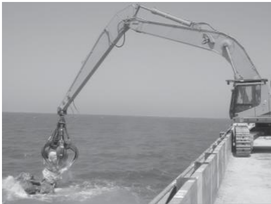
FIGURE 66: EXCAVATOR ON FLAT TOP BARGE [VAN OORD]
