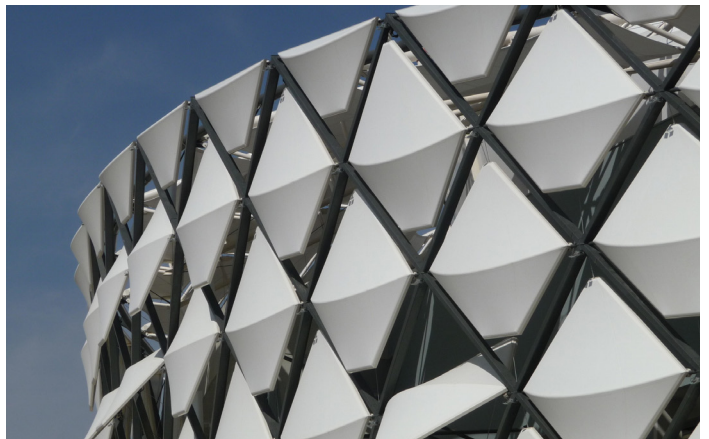
Figure 110: PTFE shading panels at the Hazza Bin Zayed Stadium. [source: Hazza Bin Zayed Stadium: MakMax Group (Taiyo Kogyo): Tensile Membrane Structures. (2020, September 06). Retrieved from https://www.makmax.com/de/applications/sports-de/hazza-bin-zayed-stadium-de/ ]
