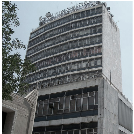
[source: OTE Telecoms Central Building, Athens. (2020, July 06). Retrieved from https://cubusengineering.gr/en/projects/commercial-building/ote-telecoms-central-building-athens/ ]
