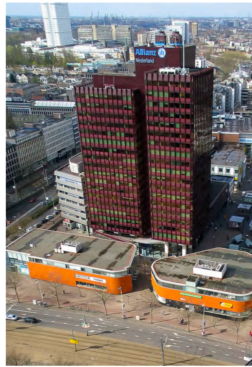
The existing situation
