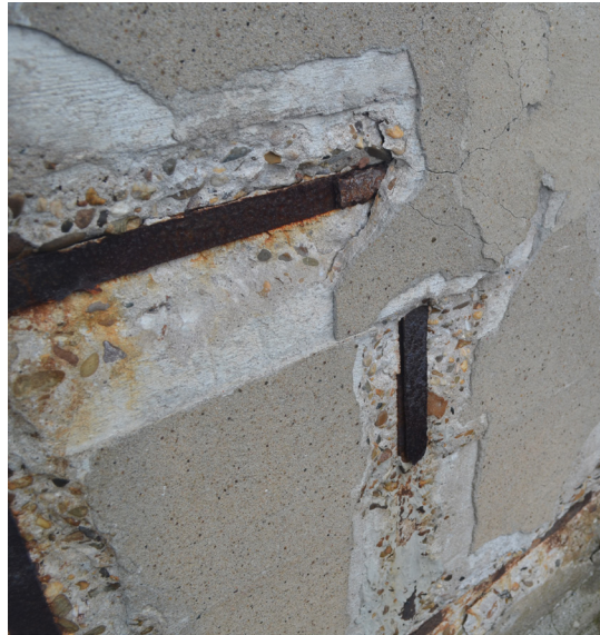
Image 2 - Wall reinforcement.
