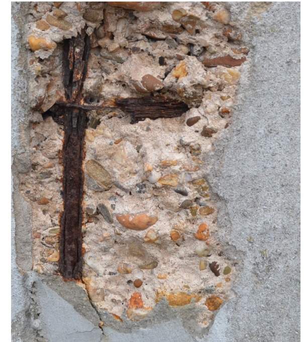
Picture of a concrete sample of the Katoenveem, Rotterdam. We observe a aggregate of rounded stone with white to brown color spectrum. Some stones have a more orange yellow character. The size of the aggregate is uneven. In the upper part possibly some air bubbles are seen.
