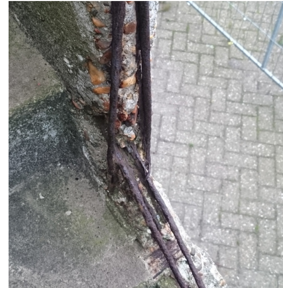
Image 3 - Reinforcement of exterior stair.
