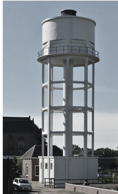
1. First open structure water tower
