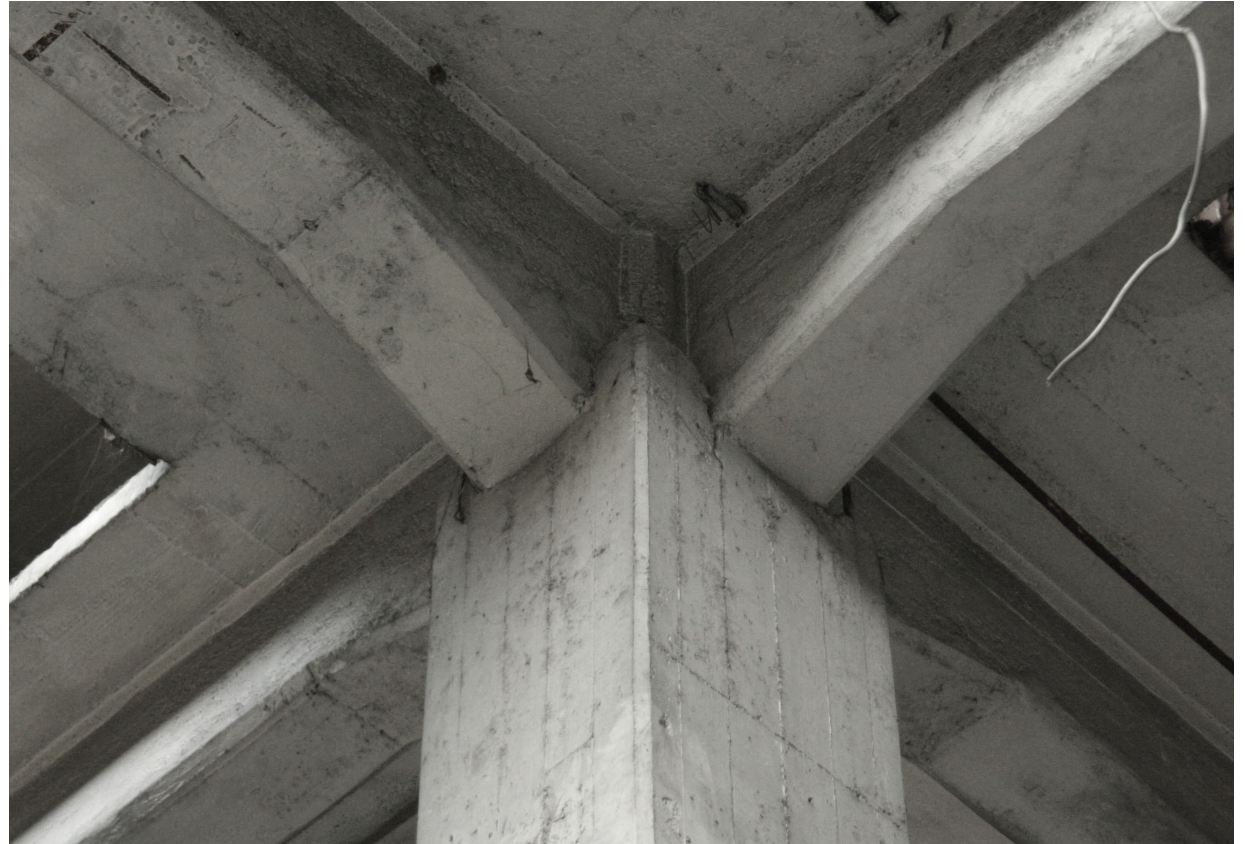
Beam column connection
