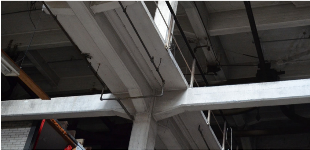
Walkway beams and non walkway beams
