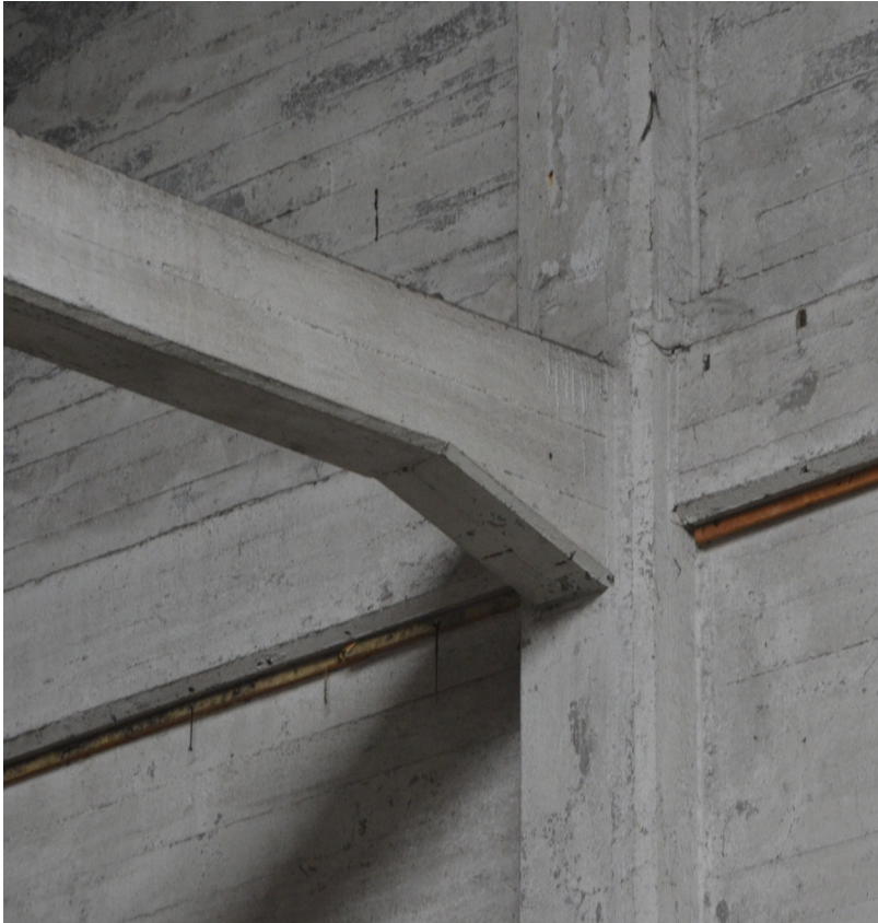
Beam compartment wall connection
