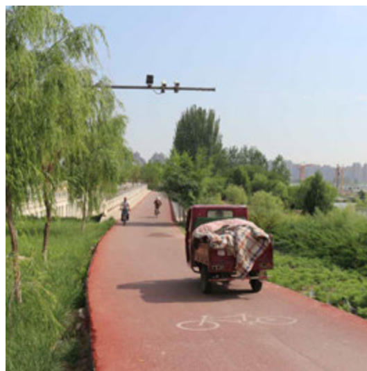
FIG. 4.77 Lack of Integration 横向连接缺乏
