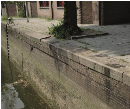
figure 4-6: deformed masonry structure by an adjacent tree (De Gijt et al., 2014)
