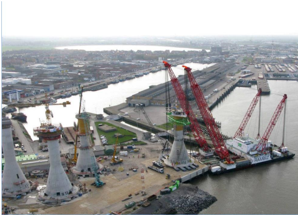
Figure A.14 - Transport of a GBS with a heavy lift vessel [48]
