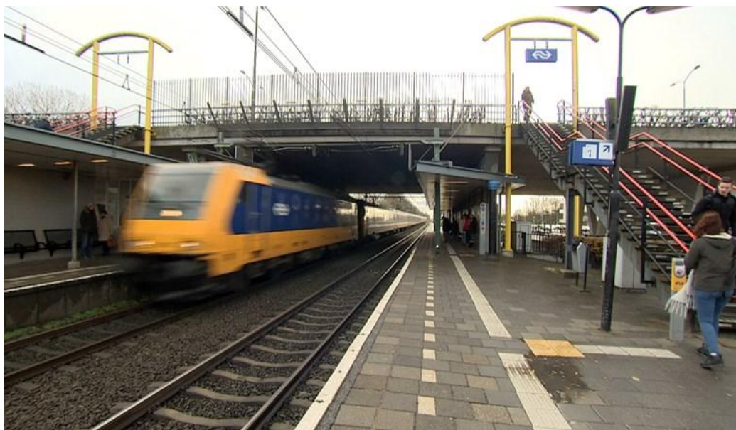
Figure 3.3: Old Delft Campus train station, named Delft Zuid station.
