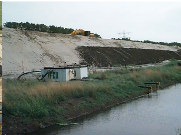
Figure 3.9: Widening of the A2 near Vinkeveen. Sand layers are gradually added to create the new embankment structure connecting Vinkeveen to the A2 [Rijkswaterstaat].
