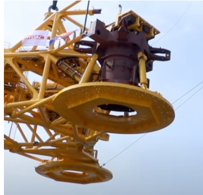
(b) Ring-shaped mud-mats with perforations and short skirts.
