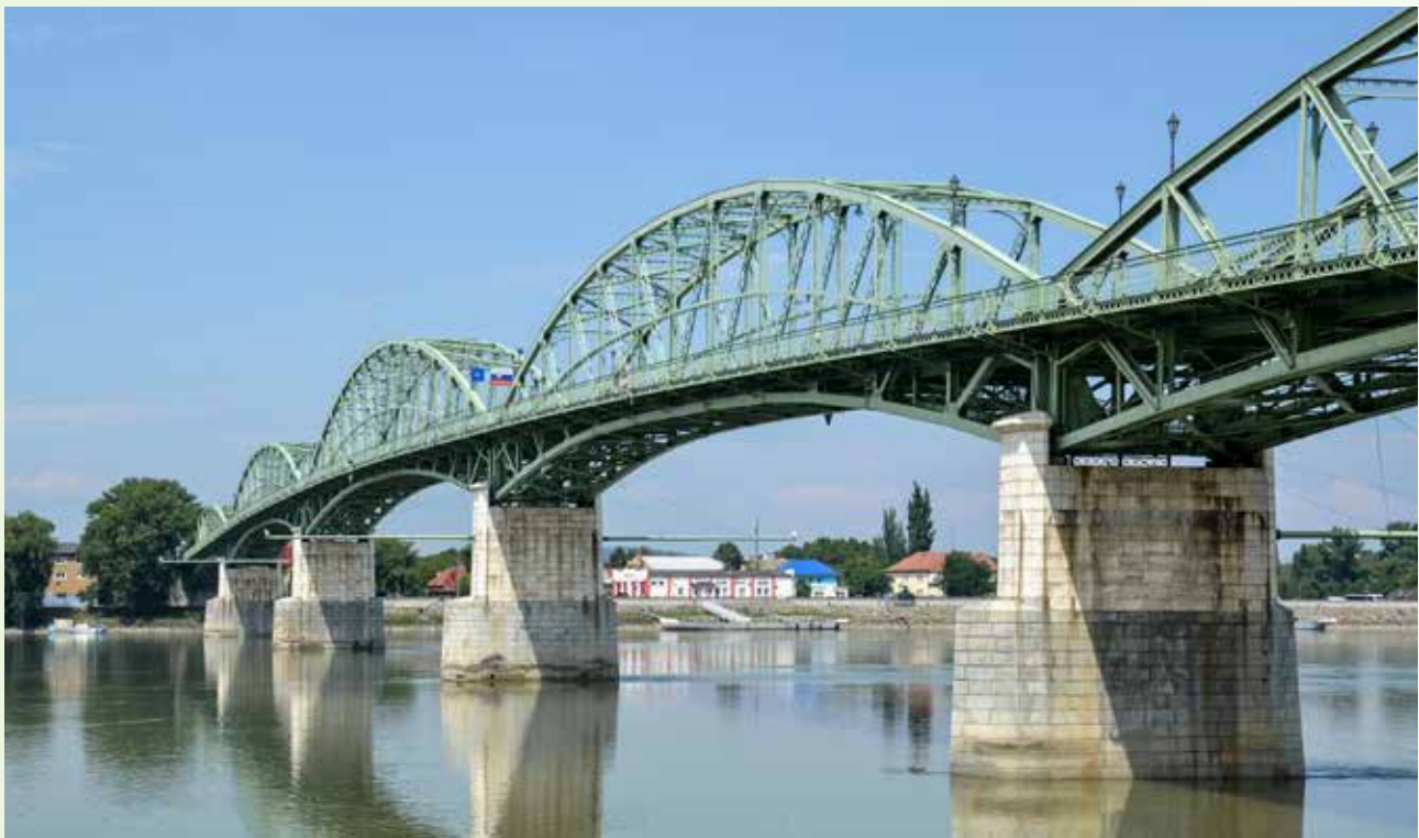
Figure 5 Mária Valéria bridge over the Danube, connecting Esztergom and Štúrovo, the site of the Bridge Guard art residency (Image: Wikimedia Commons)
