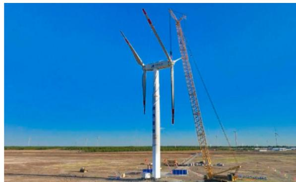
**Figure 1.14:** Dual rotor Sairui [26]
