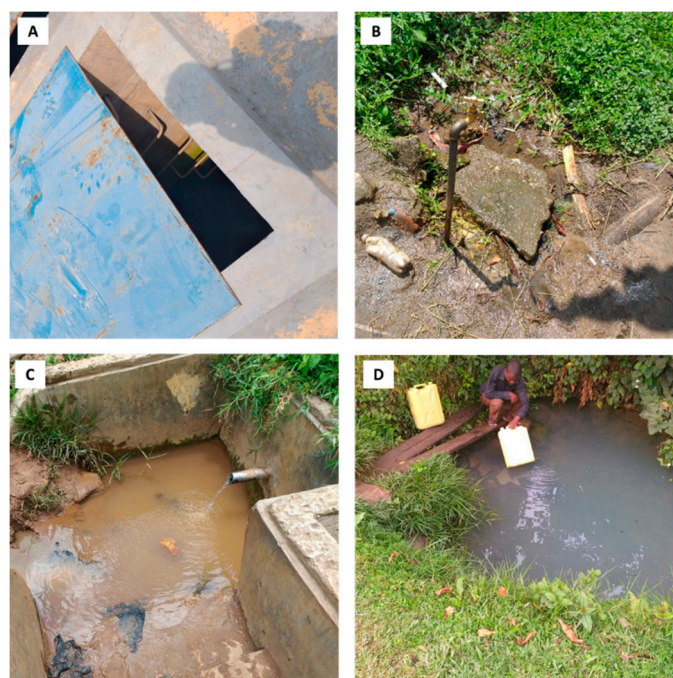
Figure 2. Photos of observable risks to water infrastructure in the study area: (A) a reservoir containing algae growth (greenish color on the inside stairs); (B) a tap stand with poor drainage; (C) a spring with an outlet pipe and inadequate drainage; and (D) an unprotected spring.
